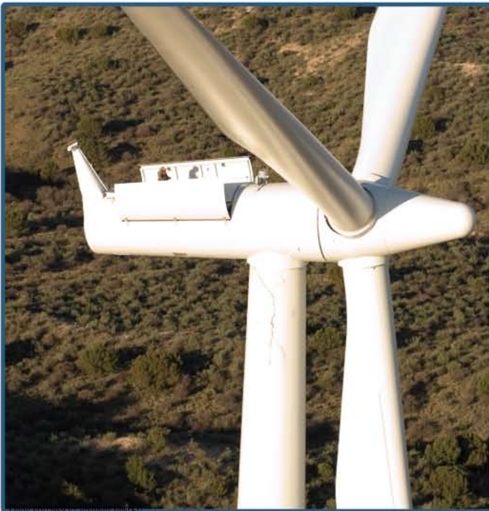
Photo provided by Siemens Energy.
